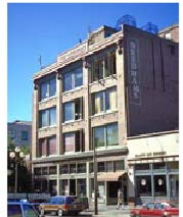
Visible communication equipment is undesirable
